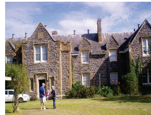
Geelong Orphan Asylum built in 1855 The first Orphanage built in Geelong.
